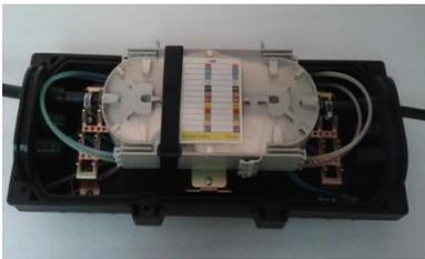
After splicing fibers and stacking trays , tie around the trays.
