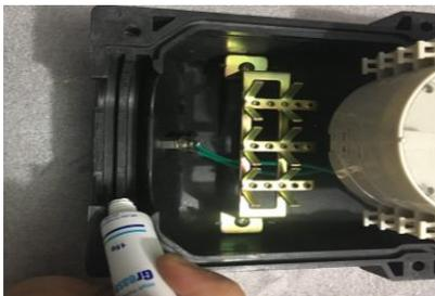
Spread the vacuum grease evenly on the gasket groove of the closure after cleaning it.
