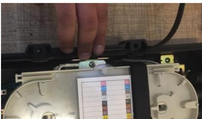
Place the side - gasket into the groove on lower case.during this step , spread **grease** on the point .where side - gasket and end - gasket meet.
